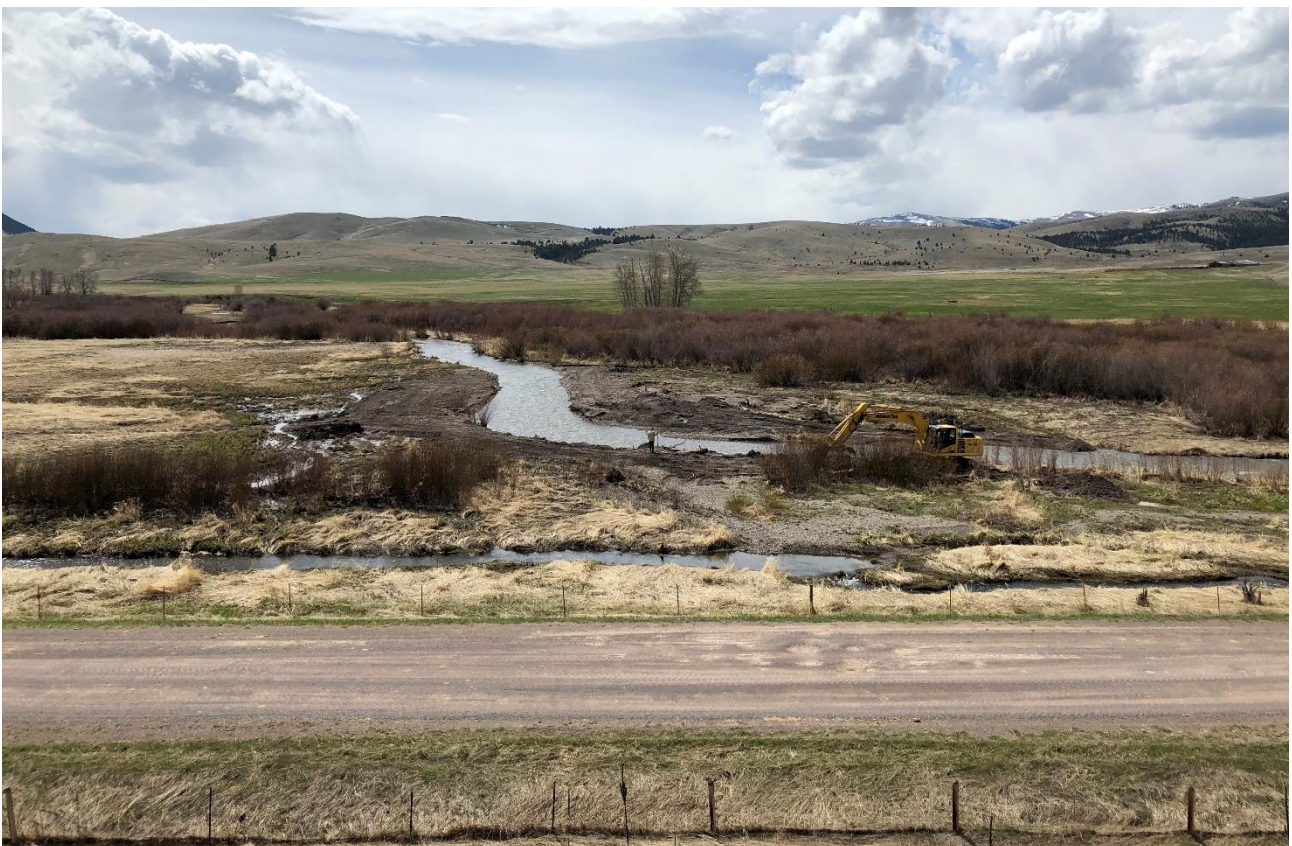
Photo 6. Little Prickly Pear Creek after 2018 flood event, during restoration. May 1, 2019.
