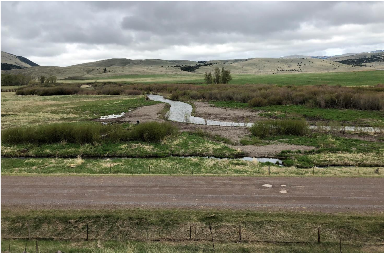
Photo 9. Little Prickly Pear Creek after 2018 flood event, after restoration. May 21, 2019.
