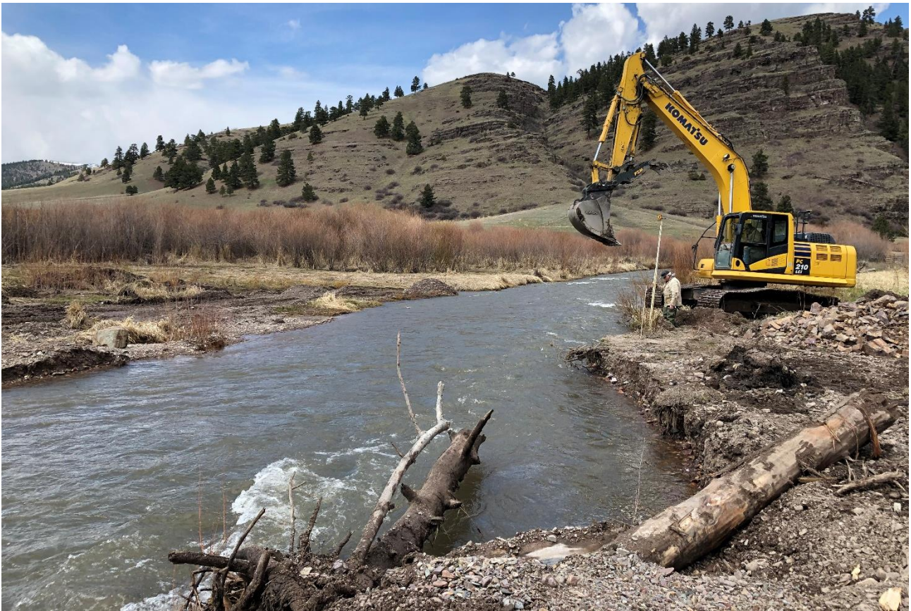
Photo 7. Little Prickly Pear Creek after 2018 flood event, during restoration. May 1, 2019.
