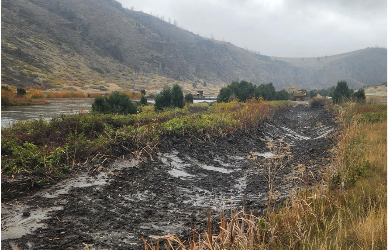
Figure 20. Photo showing side channel construction.
