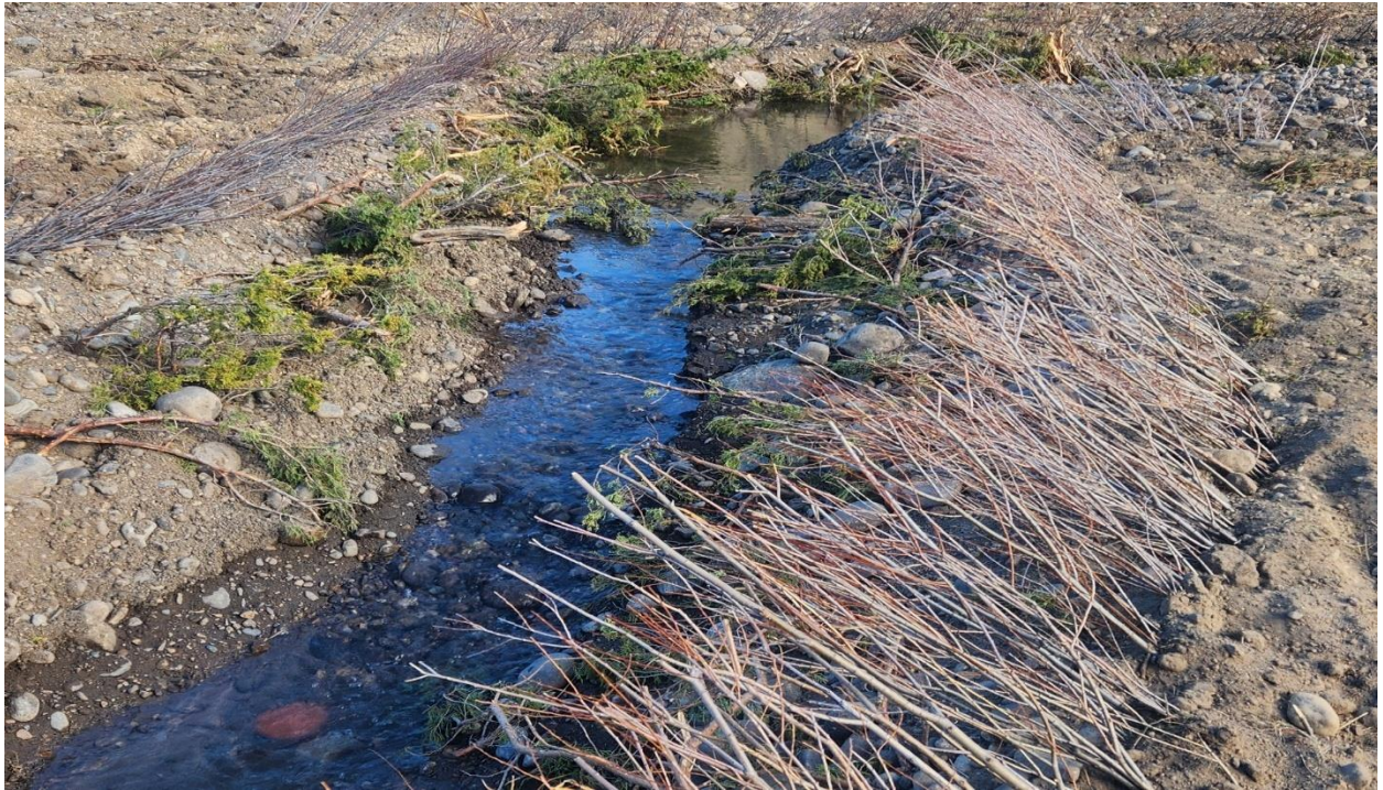
Figure 21. Photo showing a section of the completed side channel.
