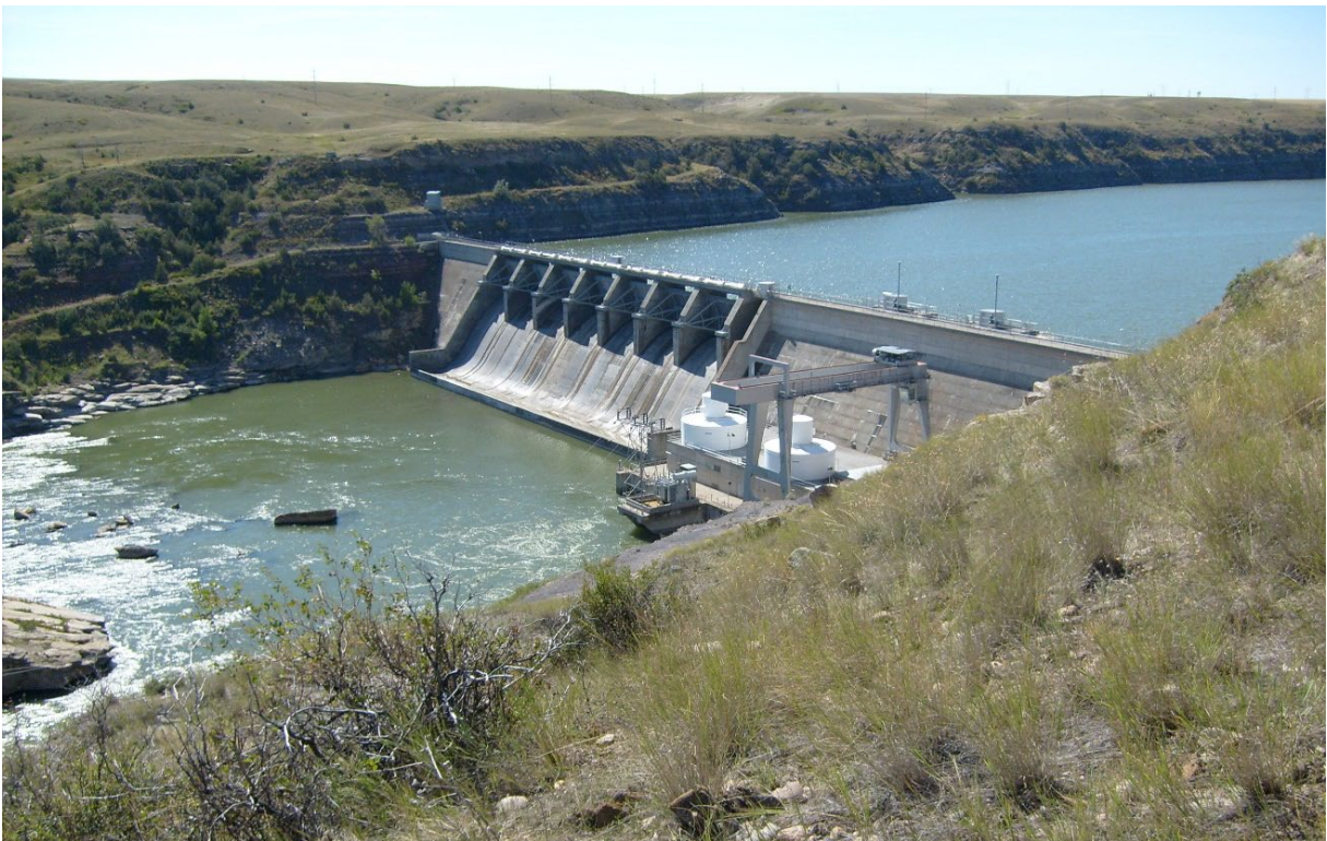
Figure 2-4: Photograph of Cochrane Dam.
