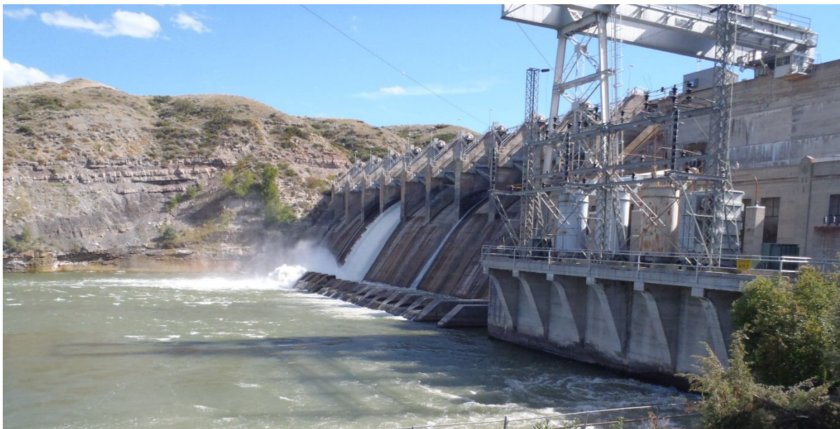
Figure 2-6: Photograph of Morony Dam.
