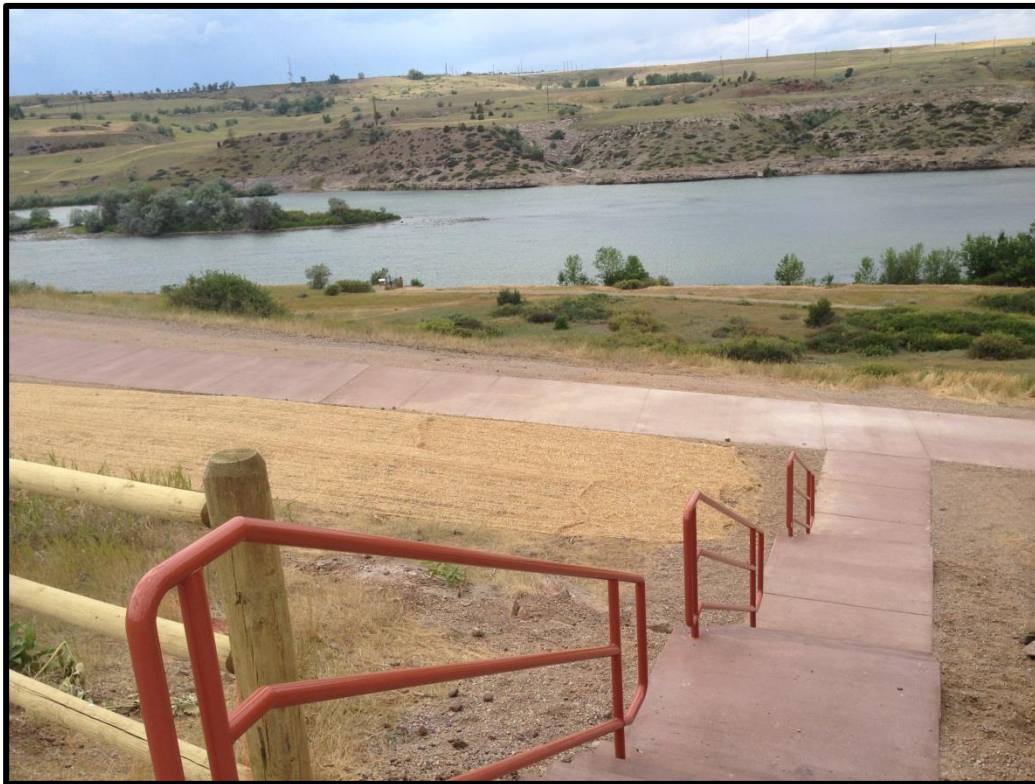
New trail surfacing and access stairway on the River's Edge Trail in Great Falls.
