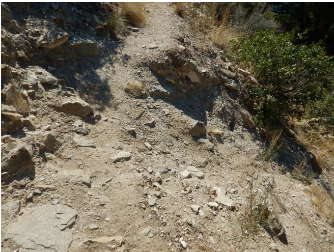
Erosion control repair section of 254
