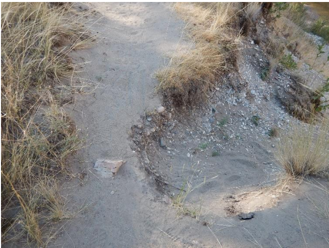
Erosion control repair section of 254
