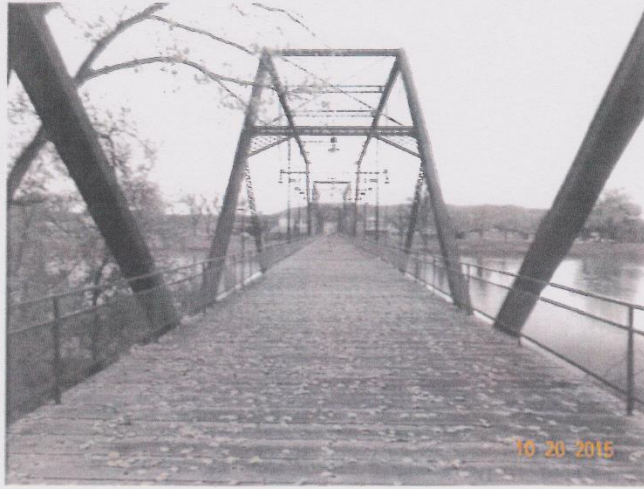
Photo 1 - General view of the bridge deck.
