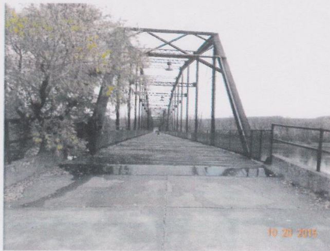
Photo 18 –View of the Span #1 with trees in contact with the downstream truss edge.
