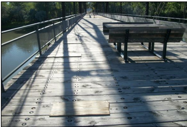
Small pieces of plywood covering holes in the deck.
