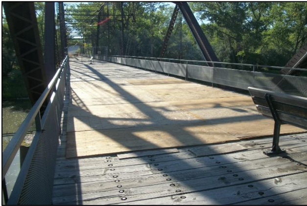
Major patching between spans.
