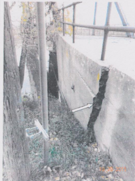
Photo 8 – View of the fractured retaining wall at Bent #1, downstream.
