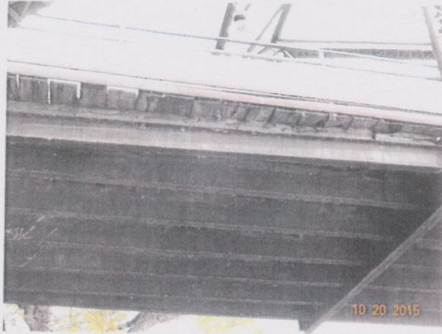
Photo 5 – View of typical deck plank attachment at Span #1 with the timber nailer attached to the steel stringer top.
