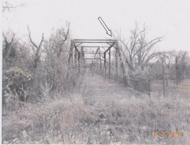
Photo 19 -View of the Span #5 with trees in contact with the downstream truss edge.
