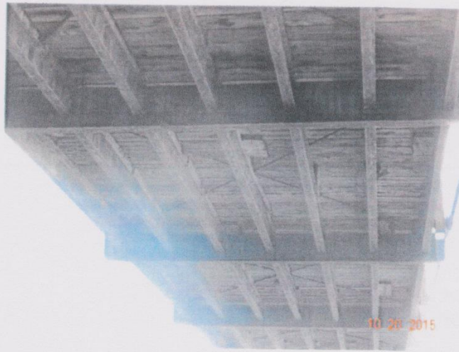
Photo 4 – View of the underside of Span #1 with past DECK failures evident.
