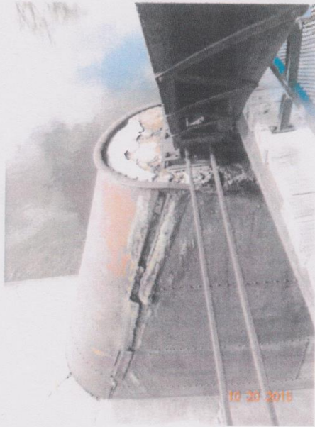
Photo 15 – Additional view of Bent #3, upstream.
