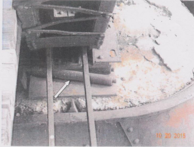
Photo 17 – Additional view of dislodged roller bearings at Bent #3, upstream.
