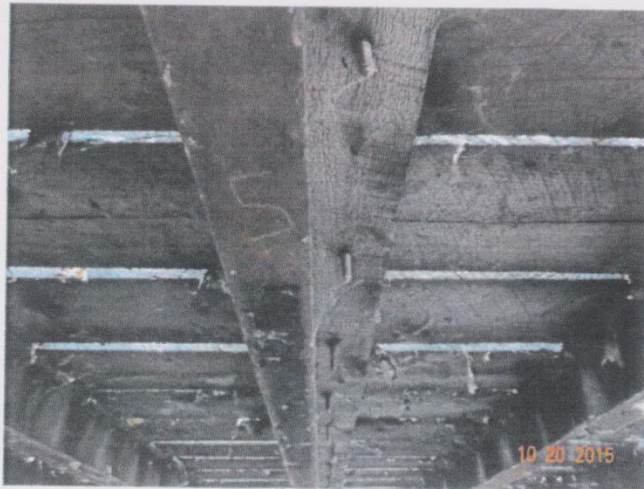
Photo 6 – View of typical deck plank attachment at Span #5 with the timber nailers attached to the steel stringer sides.
