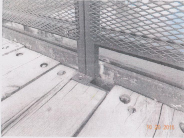
Photo 7 – View of rail connection at Span #1, upstream with a weld on the truss lower chord.
