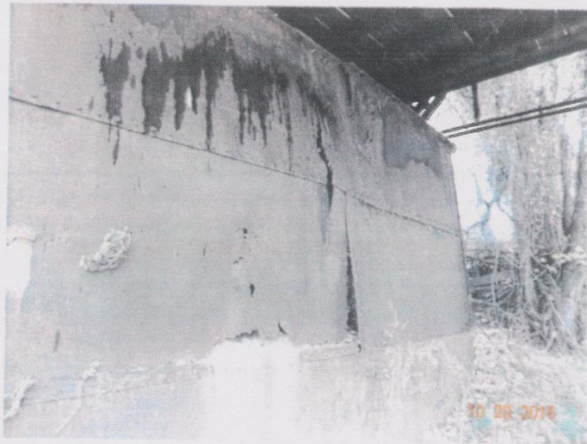
Photo 12 - View of the failed steel plate with a 12" void behind at Bent #6.
