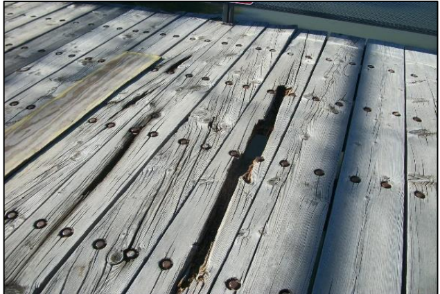
Failed decking not yet patched.
