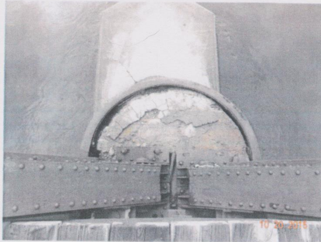
Photo 16 – View of dislodged roller bearings and poor concrete at Bent #3, upstream. Also, typical of Bent #5, upstream.
