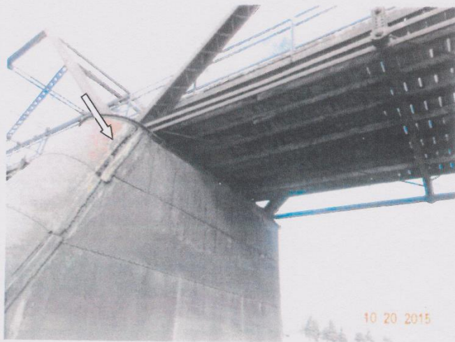
Photo 14 - View of failing steel plate at Bent #3, upstream.
