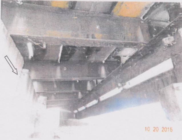
Photo 9 - View of cracked endwall at Bent #1.
