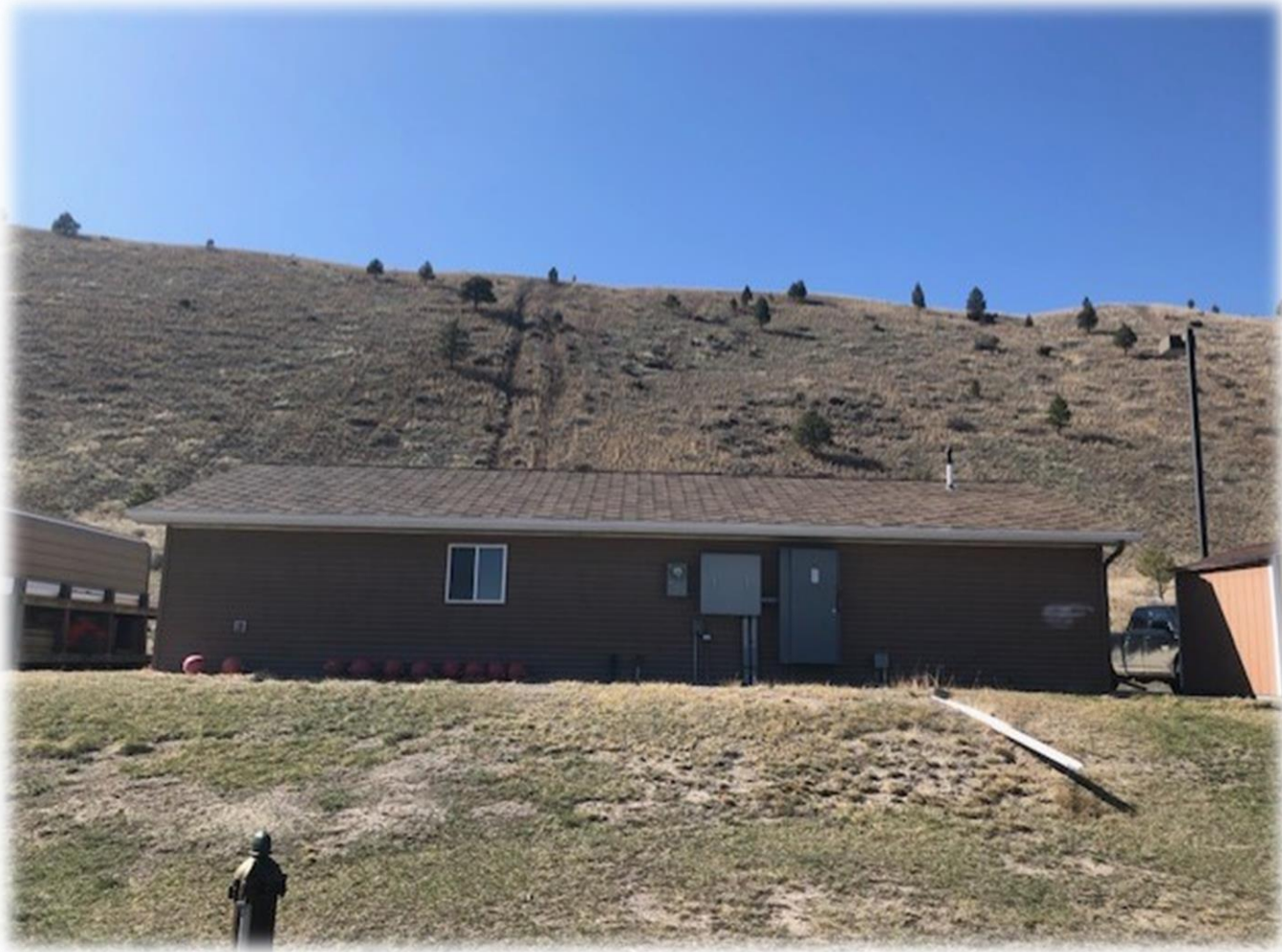
White Sandy Campground Admin Building 1
