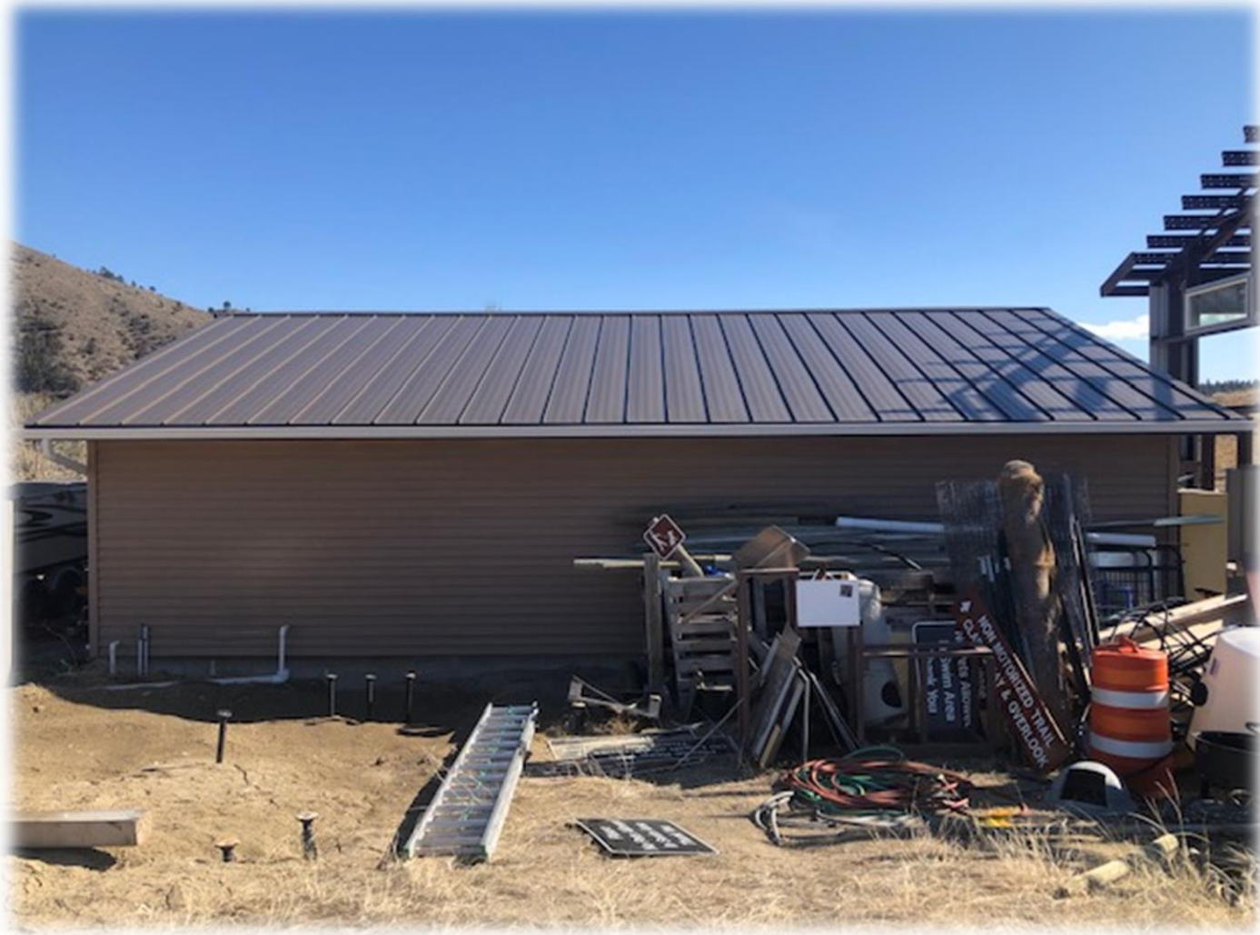
Devil's Elbow Garage Roof 1
