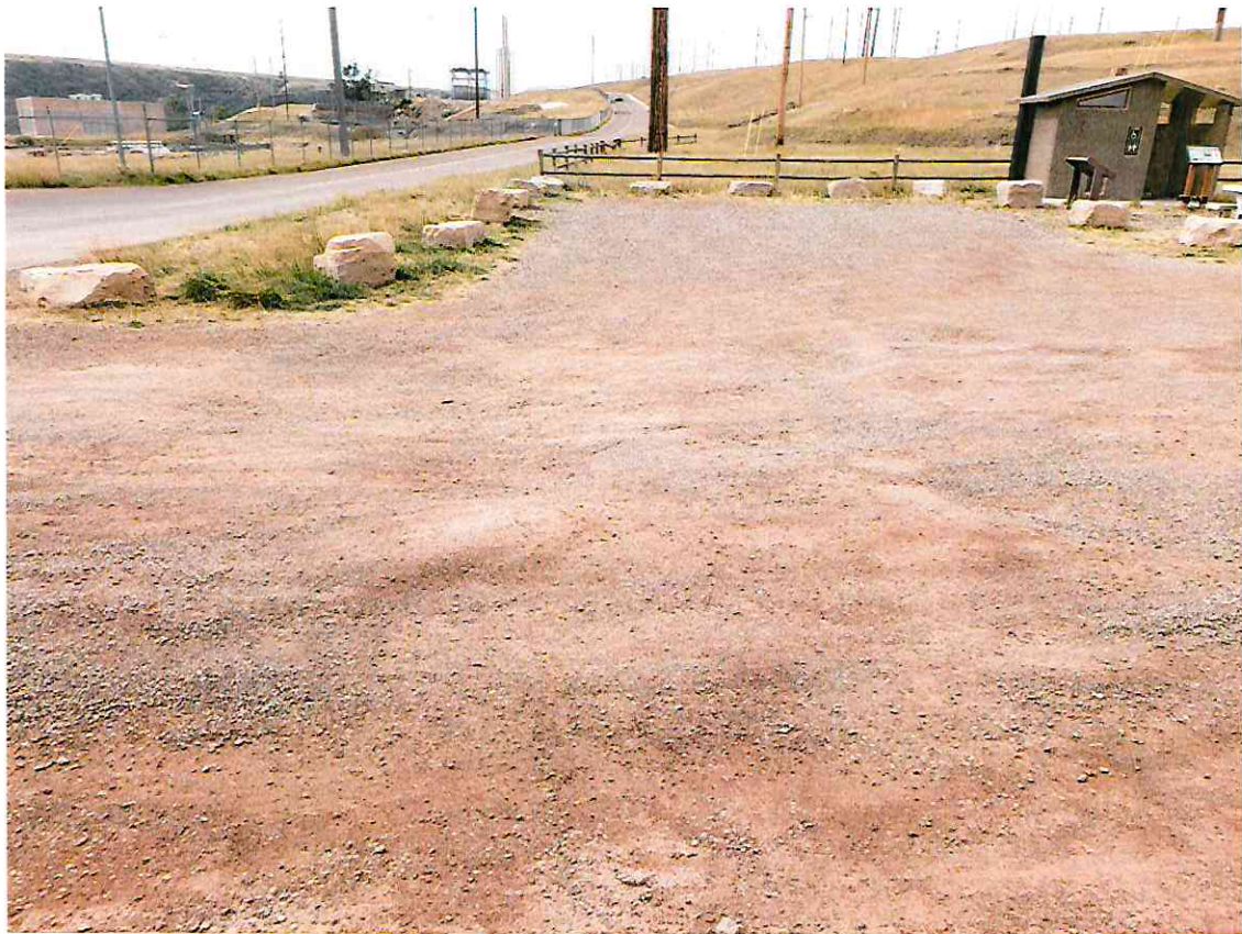
Potholes in Rainbow Trailhead
