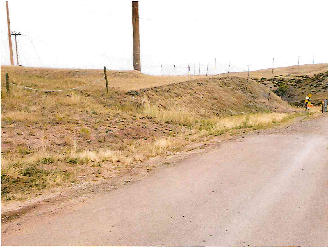
Drainage are that will be improved to the northeast
