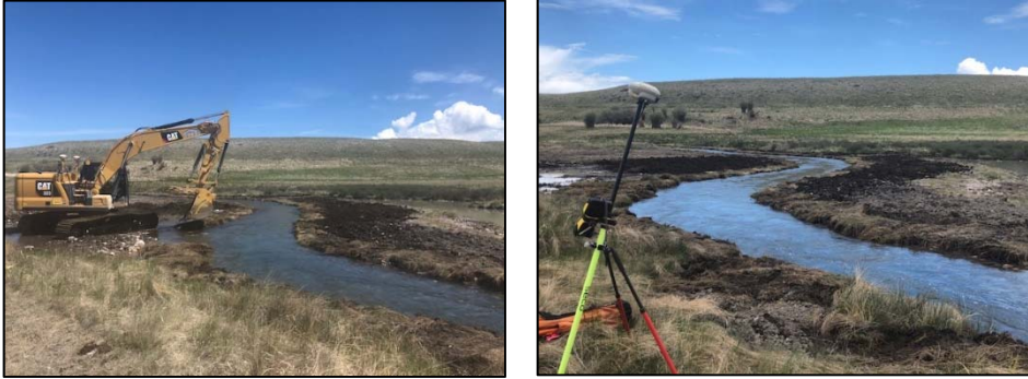
Figure 2. Construction photos from Phase 15.
