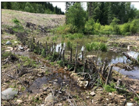
Figure 3. An example of a constructed beaver dam analog (RDG, 2019).
