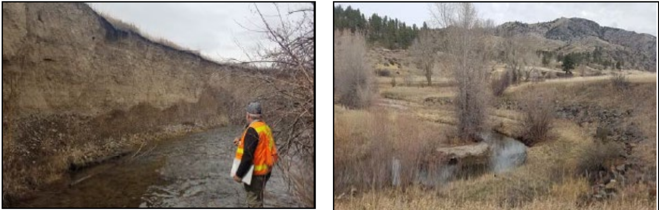
Figure 2. Pictures display channel incision and bank instability in Reach 2, rip-rap streambank modification/stabilization is common throughout the project area. Beaver Creek is listed for sediment and stream-side alteration impairments (MT DEQ).
