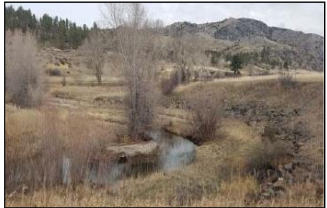
Figure 3. Pictures display channel incision and bank instability and lack of floodplain connectivity in Reach 3. Rip-rap streambank modification/stabilization is common throughout the project area, implemented in response to the 1975 flood events. Beaver Creek is listed for sediment impairments (MT DEQ).
