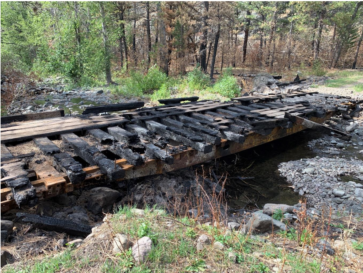
Figure 1. Bridge #2 over NF Sheep Creek with typical damage sustained during Harris Mountain Fire, September 2021.
