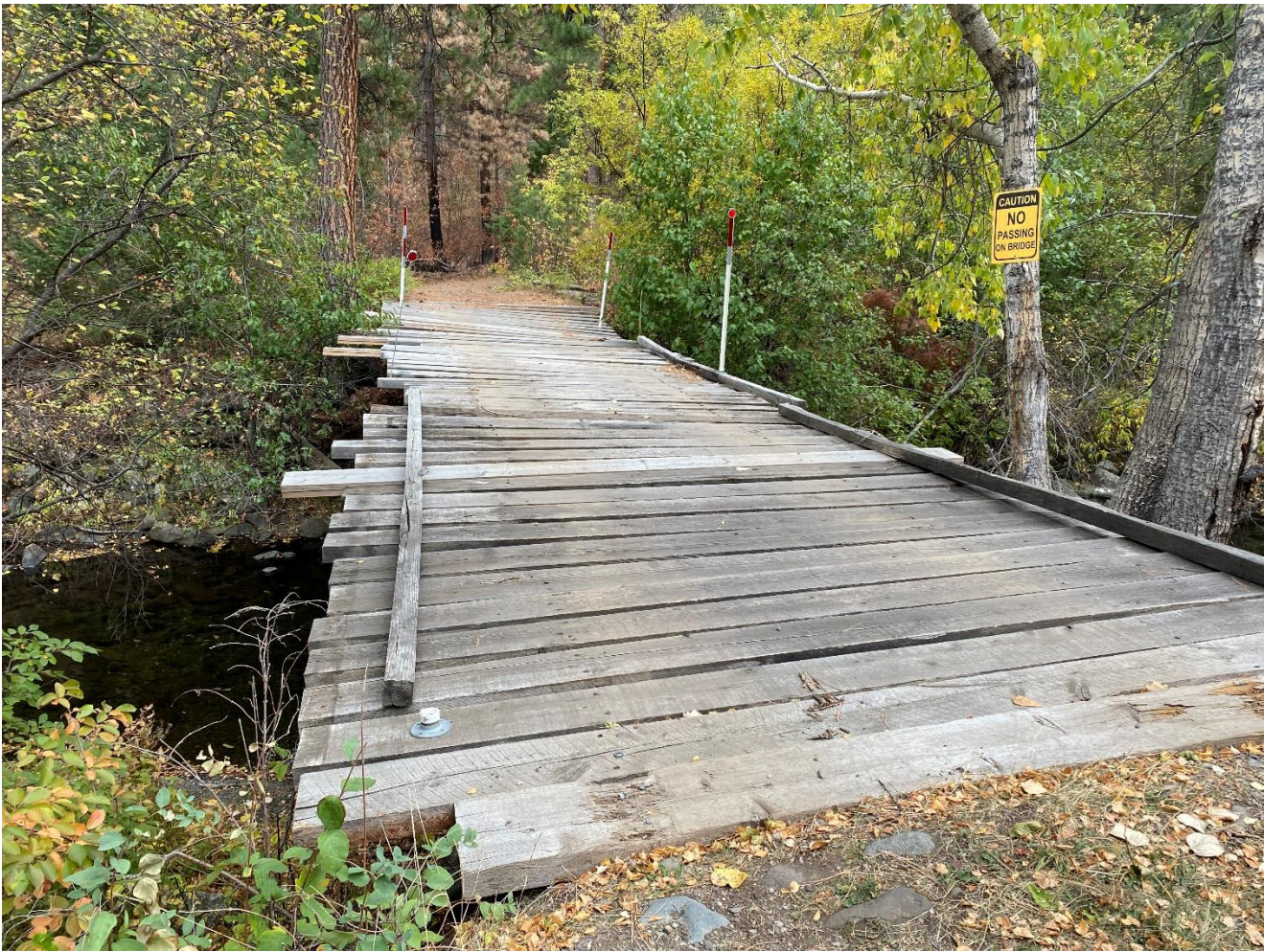
Figure 2. Bridge over SF Sheep Creek, October 2021.
