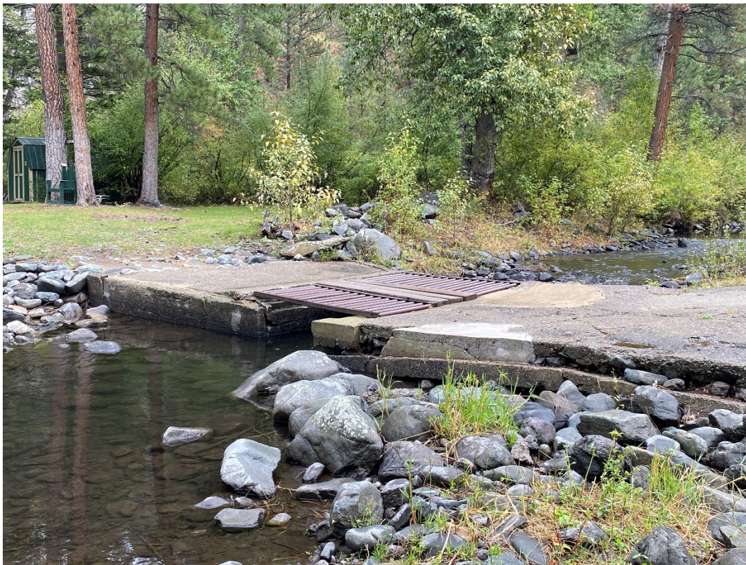
Figure 2. Ulmer ford crossing looking upstream, SF Sheep Creek, Montana.
