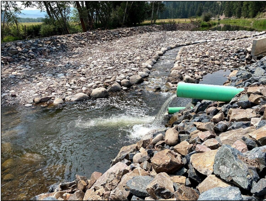
Figure 5 – Rock riffle with diversion crest at 5% slope near Hall, MT
