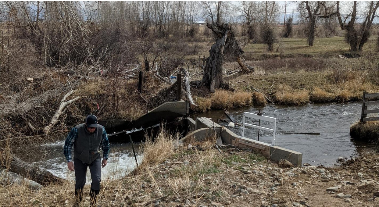
Photo 1. Diversion structure and fixed-wheel headgate (June 9, 2022; 110 CFS).
