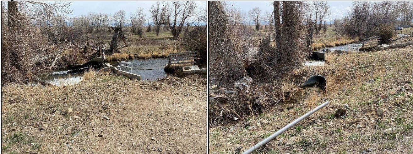
Figure 2 – Existing Diversion and Headgate Structure
