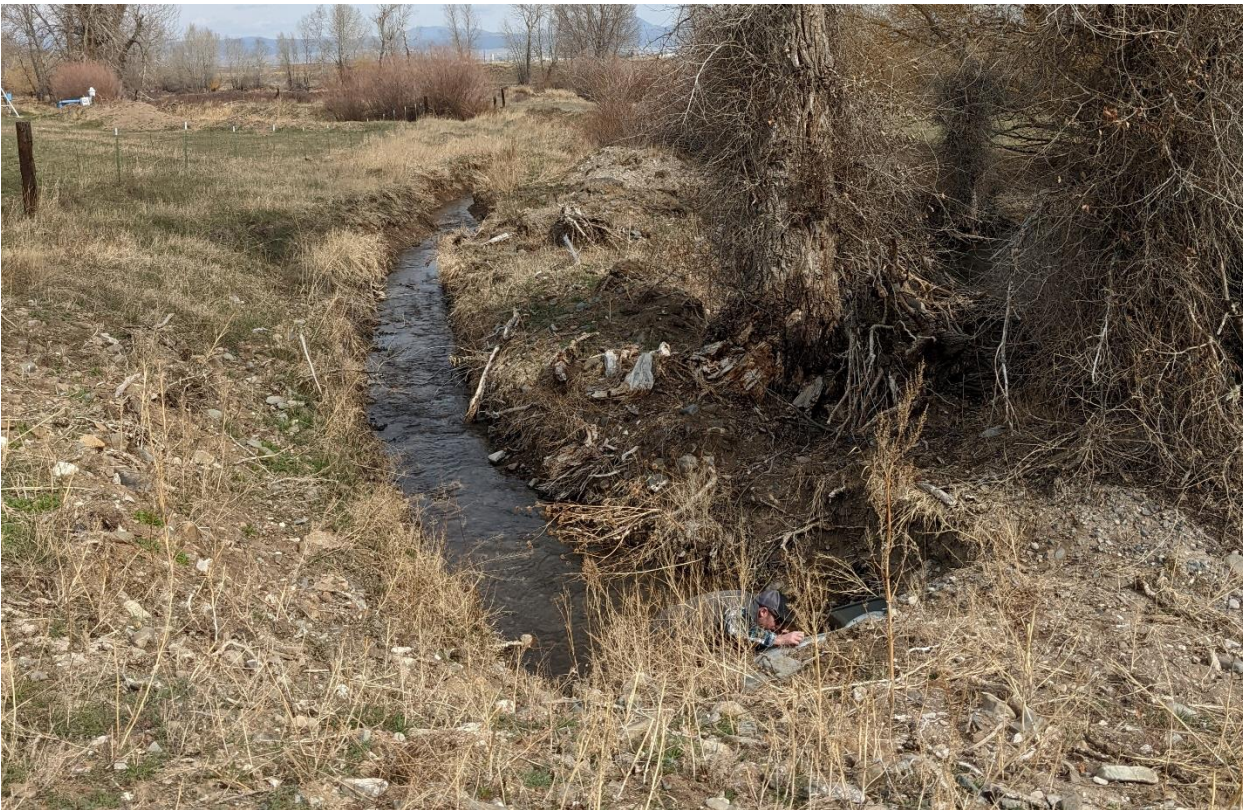
Photo 2. View of from the headgate pipe looking downstream into the irrigation canal (June 9, 2022).
