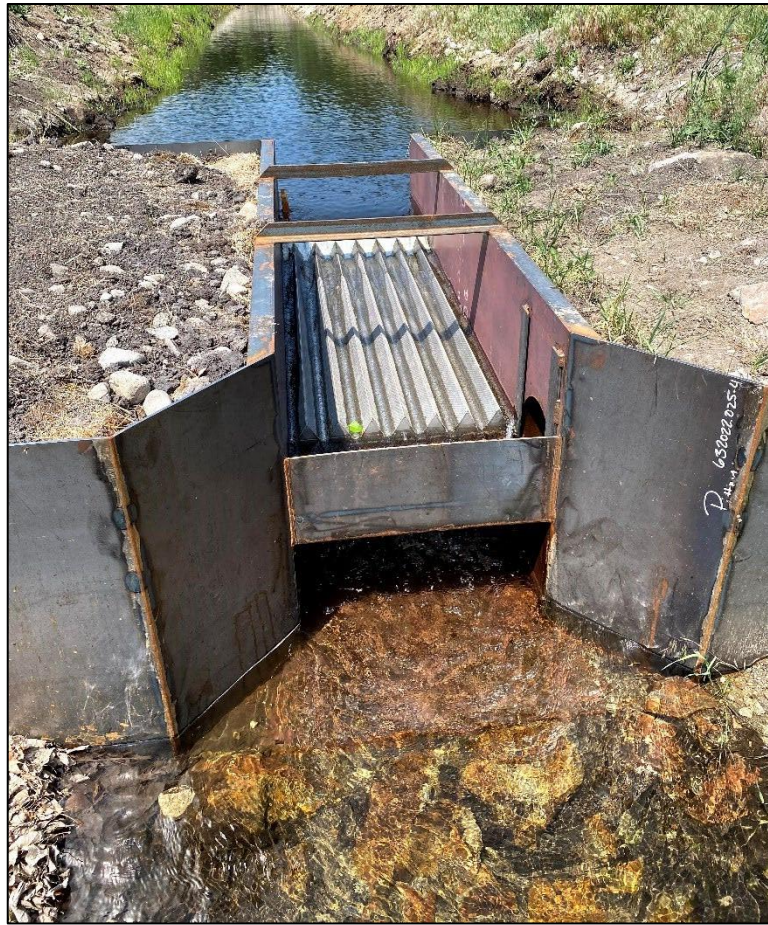
Figure 3 – Corrugated Water Screen near Opportunity, MT
