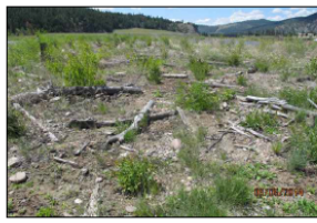
EXAMPLE OF CONSTRUCTED FLOODPLAIN ROUGHNESS
