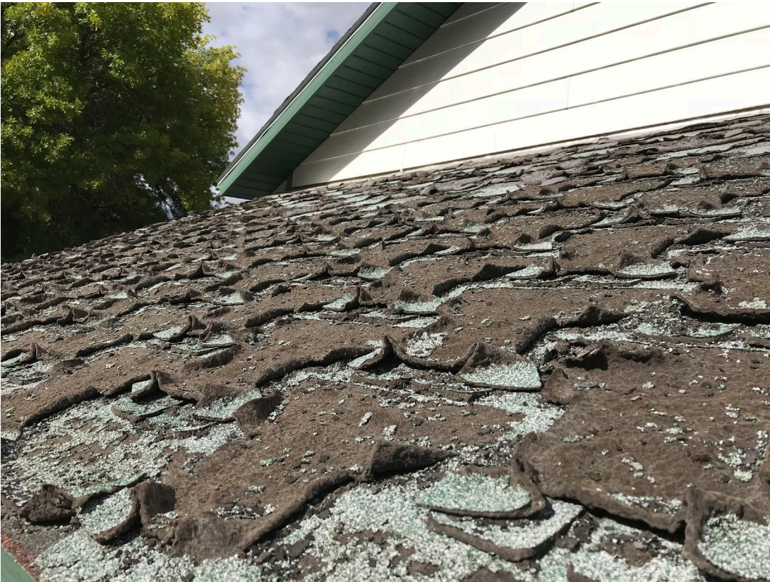
Figure 1. T-lock shingles on Holter boat house south side. October 2018.
