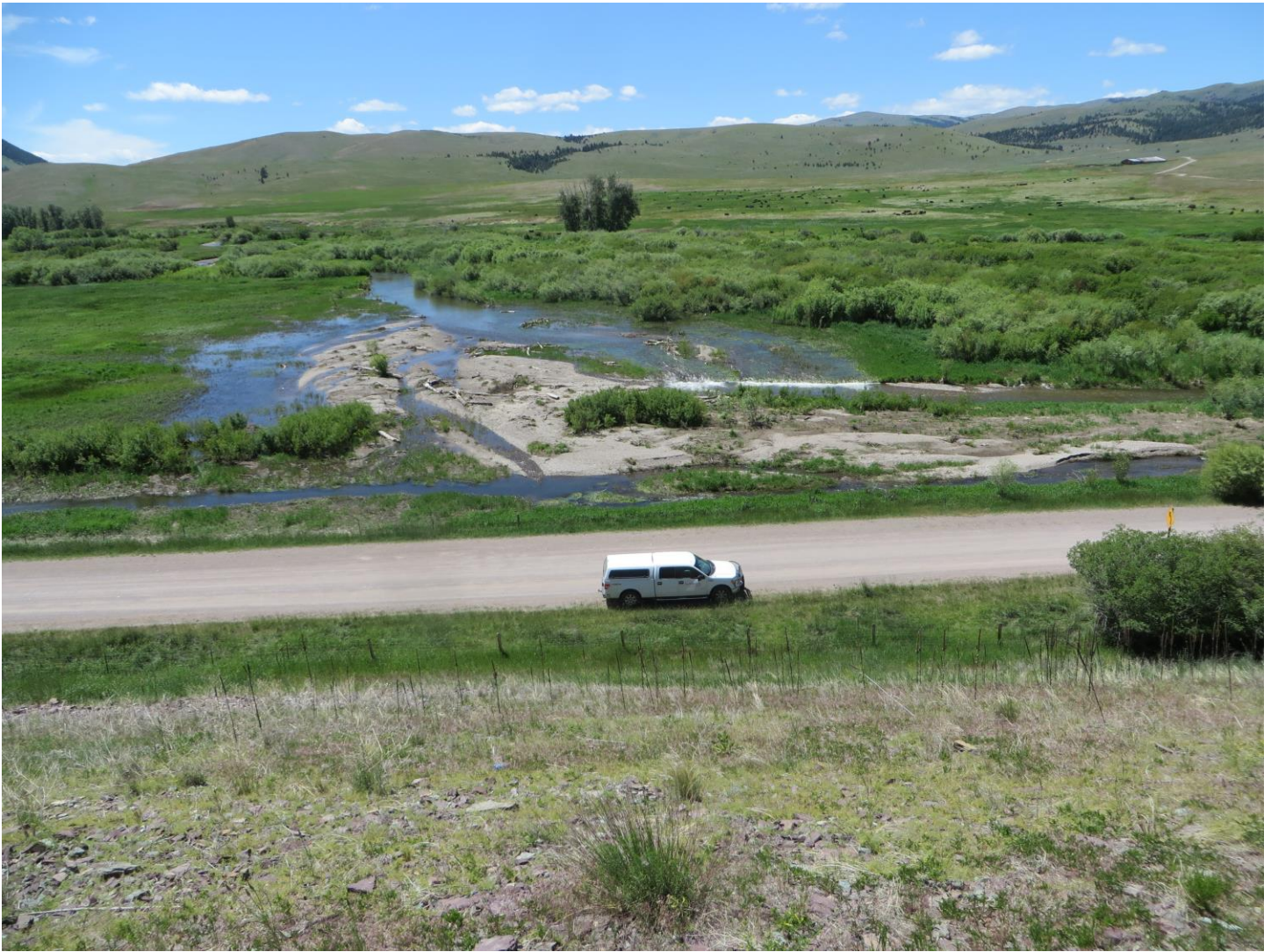
Photo 2. Little Prickly Pear Creek after flooding, Area 1, June 2018. Photo show large amount of sediment deposition, active headcut and lack of defined channel.
