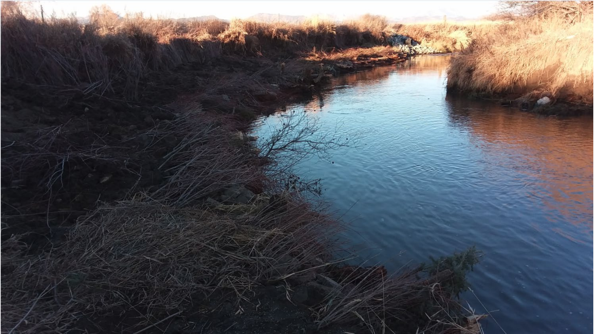
Newly constructed downstream bank. This proposal is to re-grade the inside bend (right side of photo) to increase bankfull capacity and promote point bar development.
