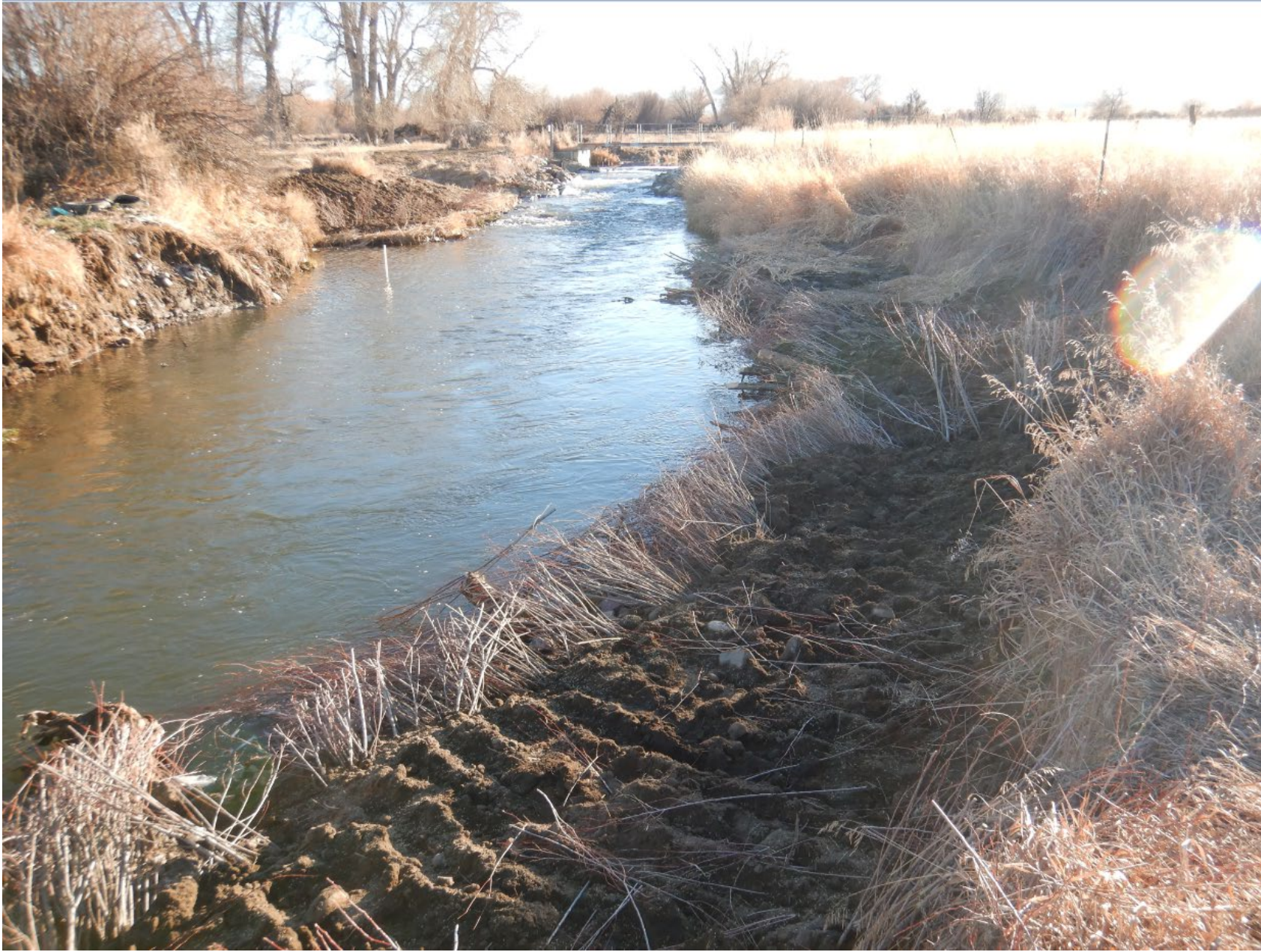
View looking upstream toward the irrigation dam. This proposal is to install Type 2 VWBF on the cut bank on the left side of the photo to reduce streambank erosion.
