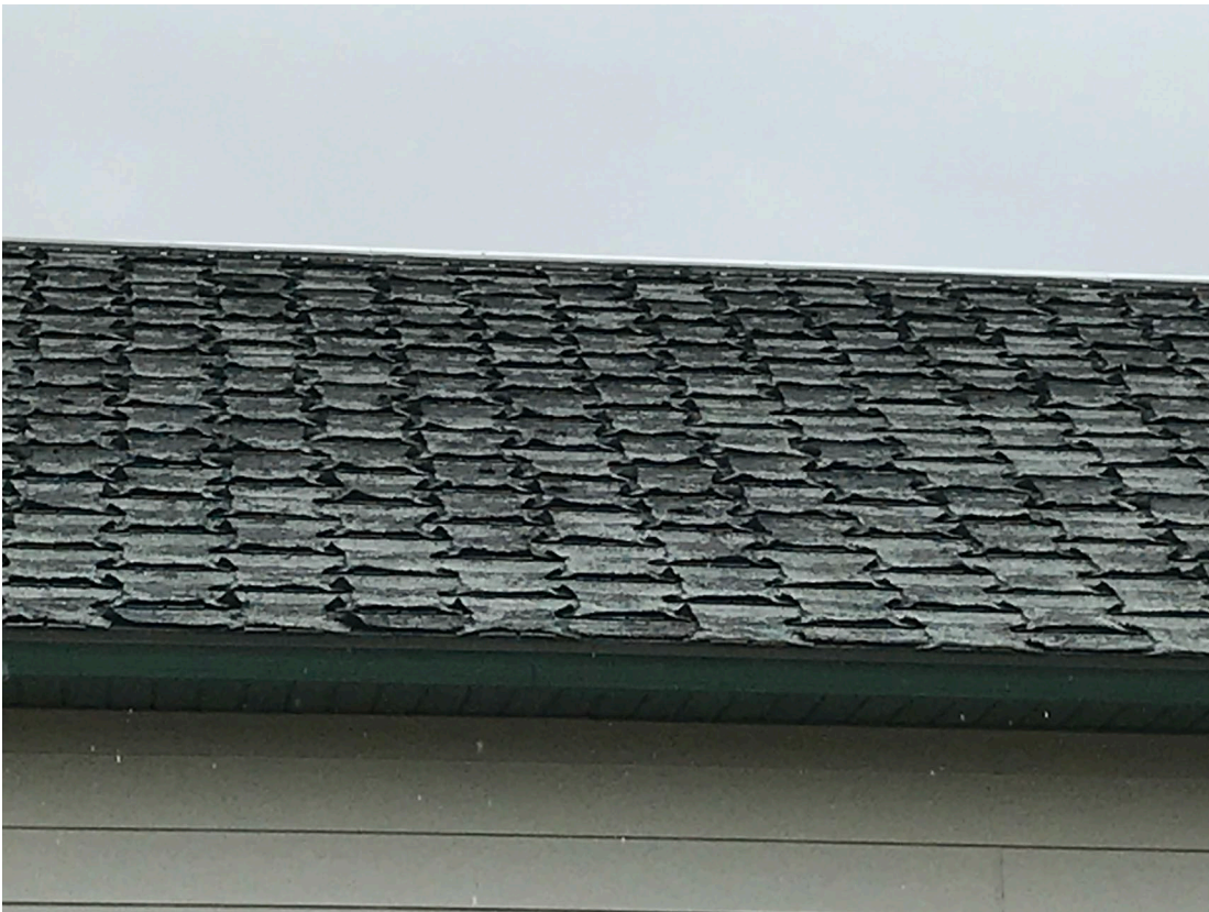
Figure 2. T-lock shingles on Holter boat house west side. October 2018.
