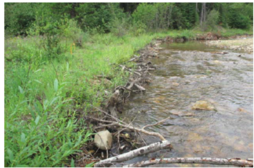
EXAMPLE OF A CONSTRUCTED VEGETATED WOOD AND BRUSH FASCINE
