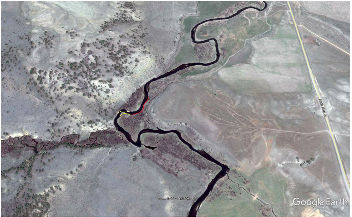
Figure 1. Aerial photo of the project area on the Smith River, downstream of Fort Logan and upstream of Camp Baker. Smith River has slowly moved closer to the Johnstone Canal is now within approximately 45 ft.
