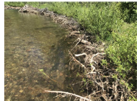
EXAMPLE OF A CONSTRUCTED VEGETATED WOOD AND BRUSH FASCINE
