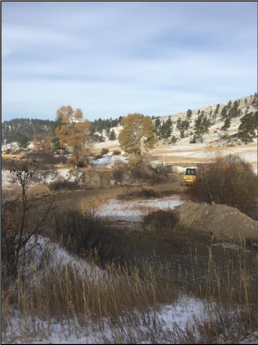
Figure 2. The River Design Group and TNT Excavating started Beaver Creek construction October 2020. Anticipated date of completion will be December 2020. Work will include reconstruction of 0.6 miles of stream channel and approximately 7 acres of reconstructed floodplain and wetland habitat. Volunteers and FS personnel have collected over 20,000 willow for streambank construction and floodplain revegetation.
