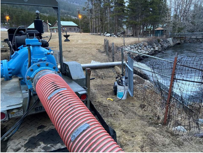
Mystic weir rebuild and dewatering.
