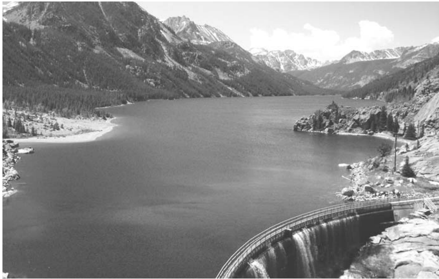
Mystic Lake in Montana is part of the 10-MW Mystic Lake hydroelectric project. Owner PPL Montana used the new integrated licensing process to prepare an application to relicense the project. PPL filed the final application with the Federal Energy Regulatory Commission in December 2006.
