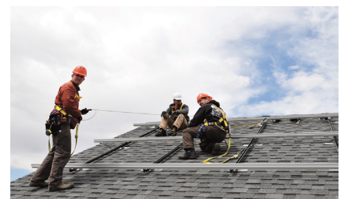
Rails/Racking Attached to the Standoffs
