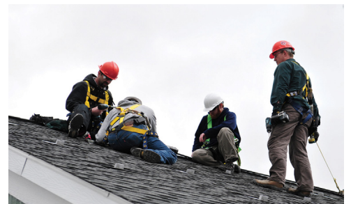
Array Standoffs Attached to the Roof's Substructure
