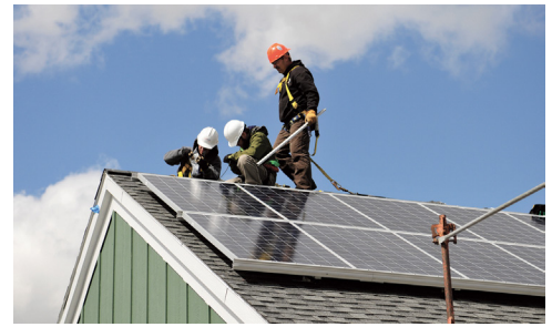
Modules Attached to the Racking
