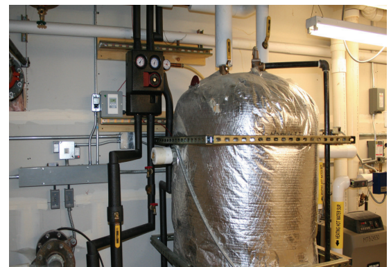
Custom Solar Hot Water Tank
