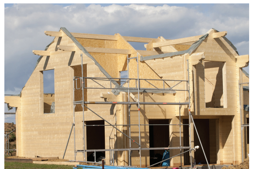
Passive Solar House Under Construction
