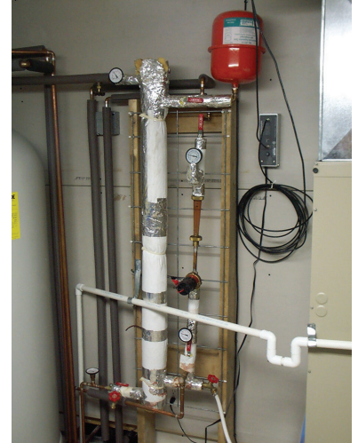
Solar Hot Water Components
