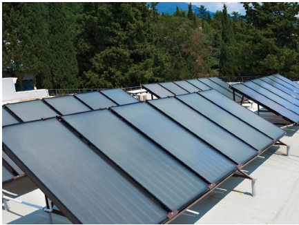
Flat Plate Collector
