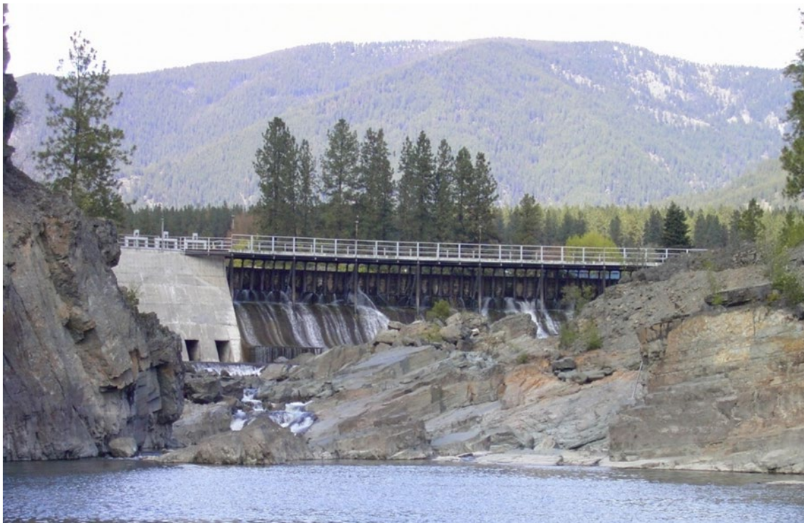
Photograph 1-3. Dry Channel Dam.
