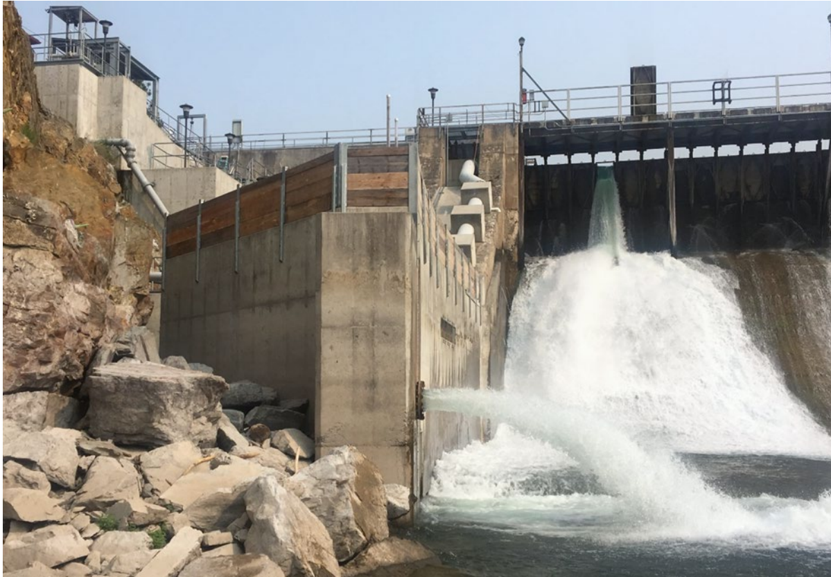
Photograph 3-6. View of attraction flows provided by HVJ and partial panel opening at the Main Dam spillway.
