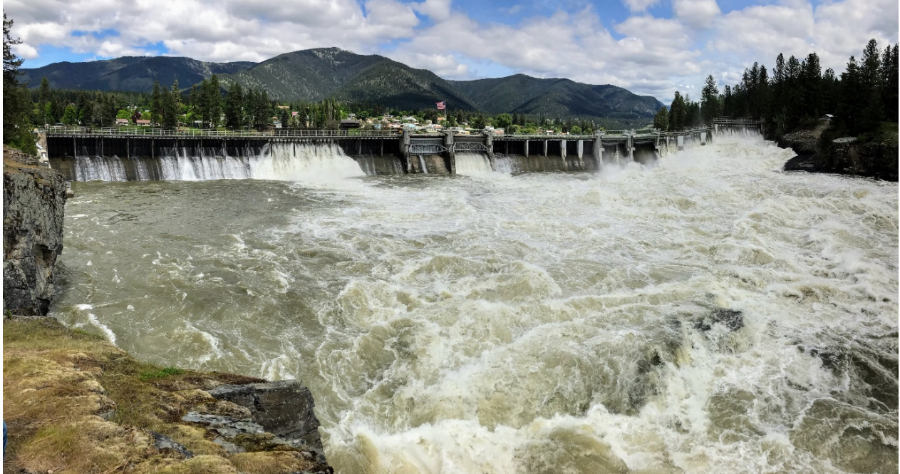
Photograph 3-7. May 23, 2019 flows 47,000 cfs. Note new radial gates on left bank (right side of photograph). Photo credit: J. Hanson.
