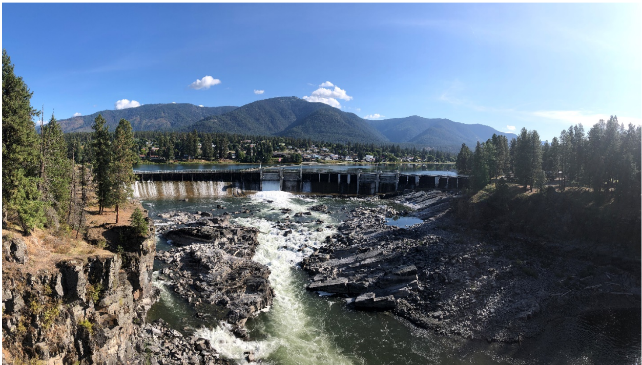
Photograph 1-2. Thompson Falls Project Main Channel Dam, with the new radial gates. Photo credit: K. Bergstrom.
