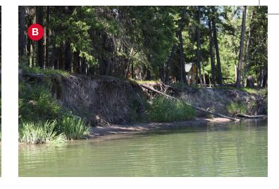
This widely used method of stabilizing reservoir banks features sloping bank down to a placed rip rap toe. While effective, this method provides little instream habitat.
