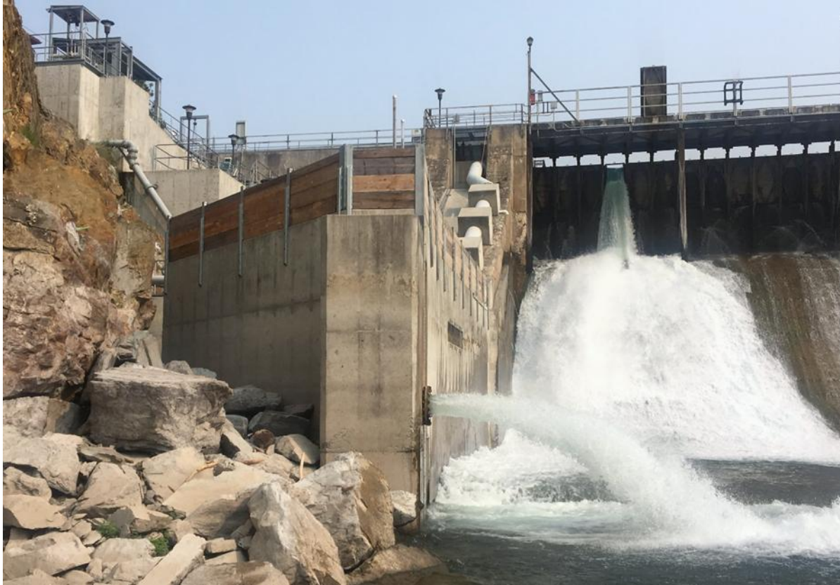
Figure 2-5. Ladder Entrance – View from downstream, showing High Velocity Jet in use
