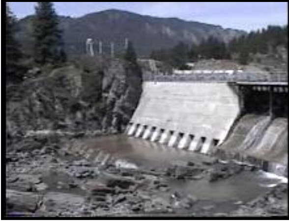
Photo 4. Dry Channel Dam at Thompson Falls, low flow.
