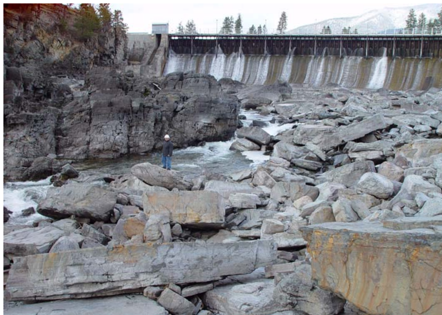
Figure 4 – Steep center thalweg and “falls” roughness.
