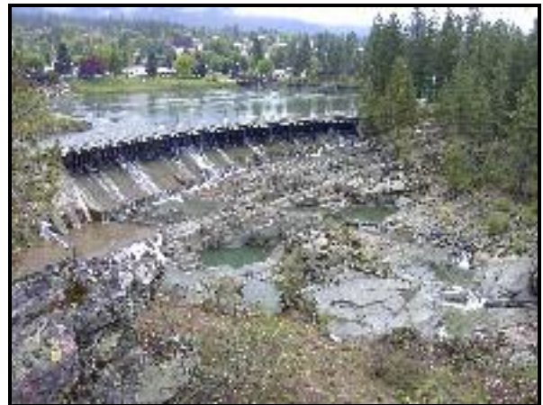
Photo 7. Dry Channel Spillway, from above.
