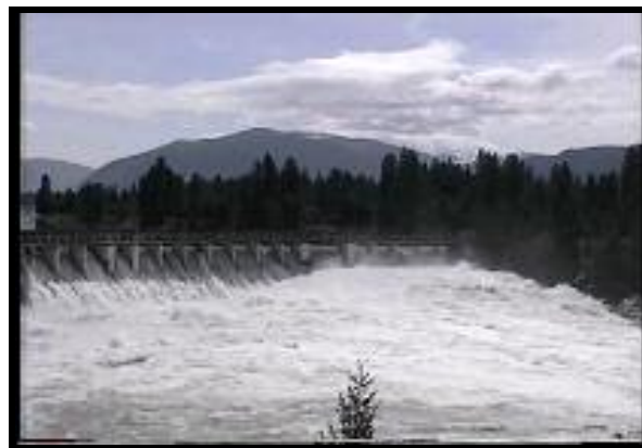
Photo 3. Main Dam Spillway at Thompson Falls, high flow (June 10, 2002, total river flow approximately 77,000 cfs).
