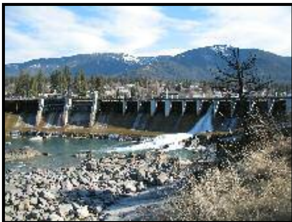
Photo 2. Main Dam Spillway at Thompson Falls, low flow (March 20, 2006).
