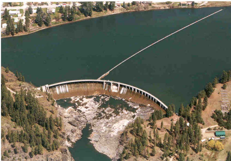
Figure 3 – Aerial photo of Main Dam Spillway.
