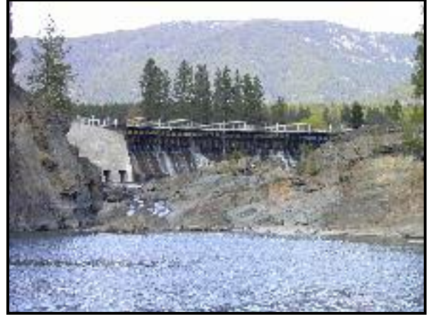
Photo 6. Dry Channel Spillway, looking upstream.
