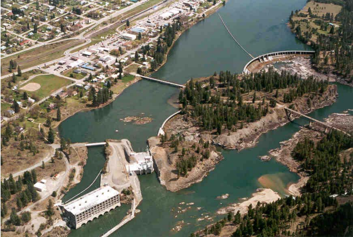
Figure 2. Aerial photo of the Thompson Falls Project, looking upstream. The Main Dam spillway is in upper right and full height fishway will be located on the right abutment of the Main Dam (looking downstream). Photo courtesy of PPL Montana.
