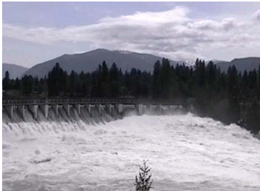
Figure 4. Photos of Main Dam Spillway at Thompson Falls at low flow (upper photo from left bank; March 20, 2006) and high flow (lower photo from right bank; June 10, 2002, total river flow approximately 77,000 cfs).
