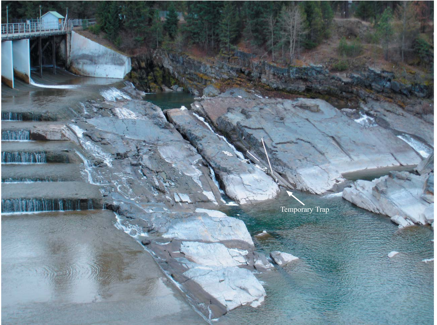
Main Dam Spillway - Left Abutment
