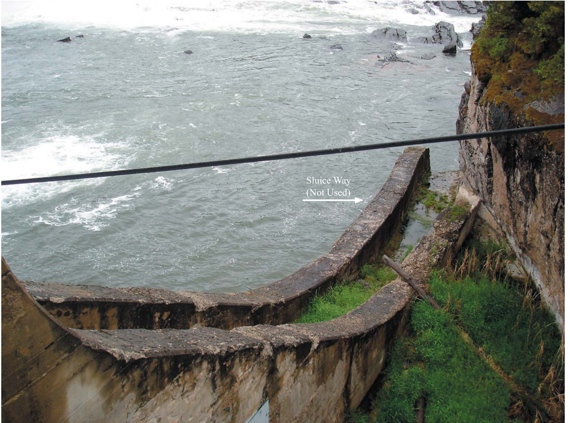
Main Dam Spillway - Right Abutment
