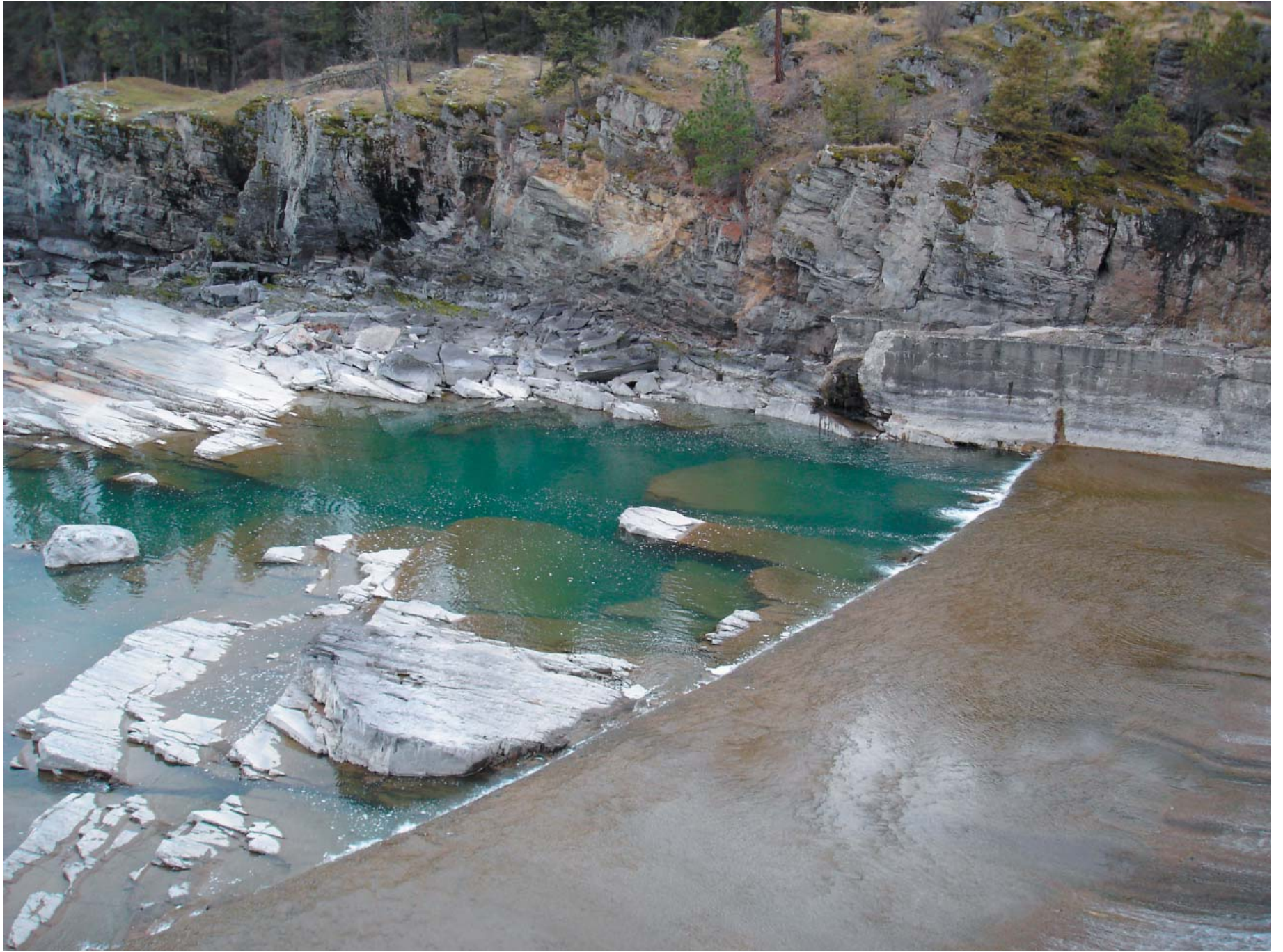
Main Dam Spillway - Right Abutment
