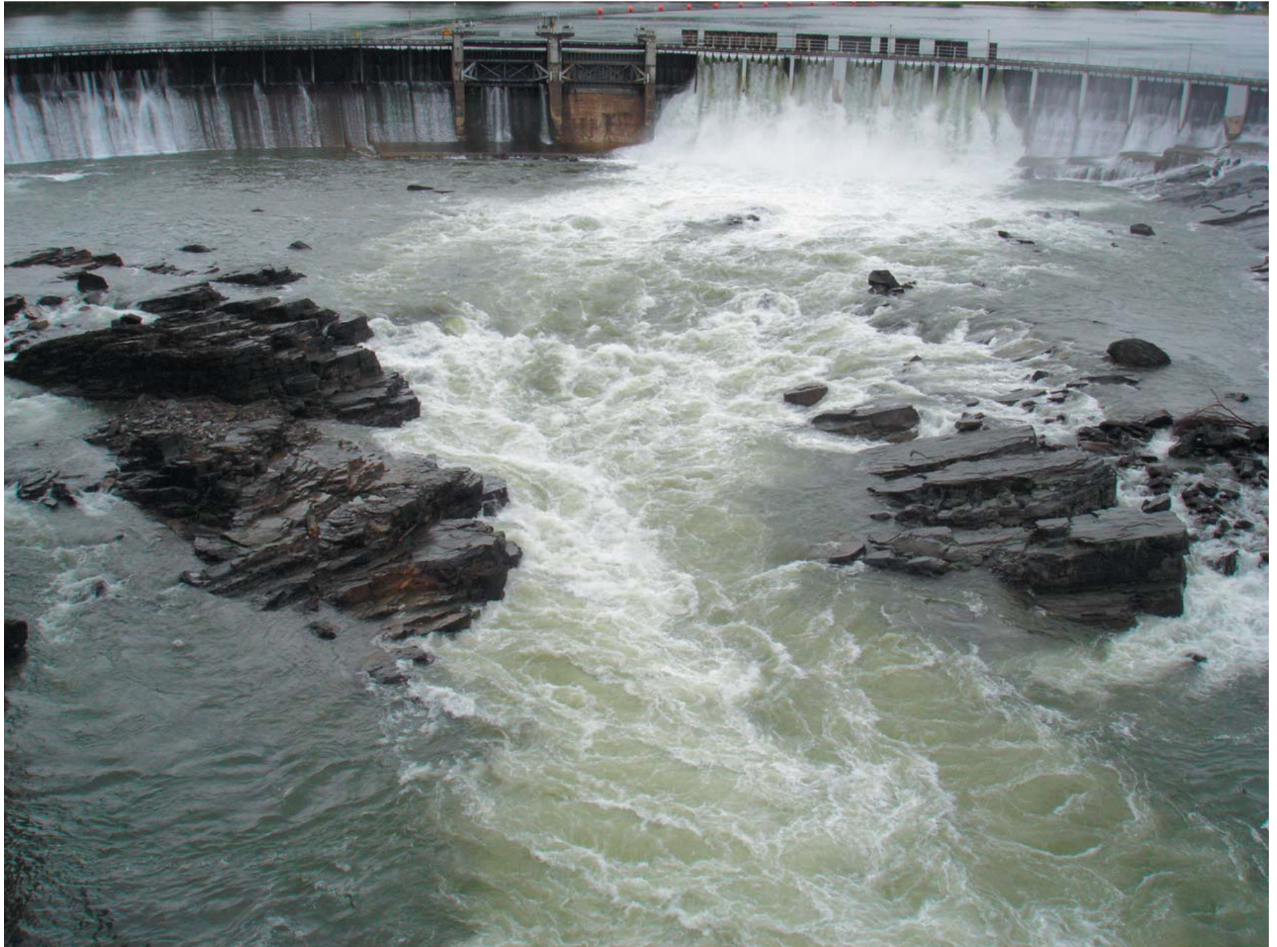
Main Dam Spillway with 6,000 CFS Spill
