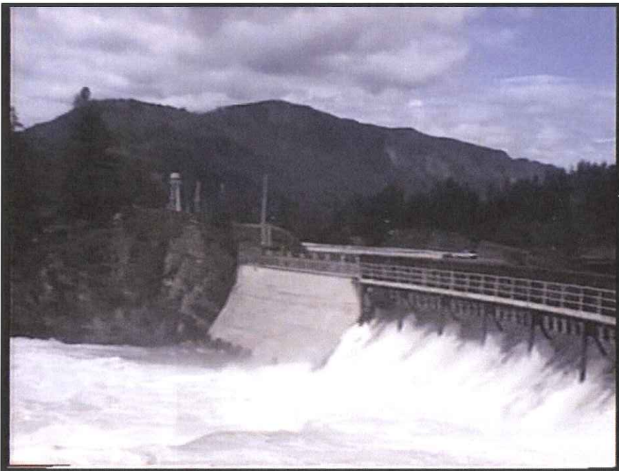
Photo 5 Dry Channel Dam at Thompson Falls, high flow (June 10, 2002, total river flow approximately 77,000 cfs)
