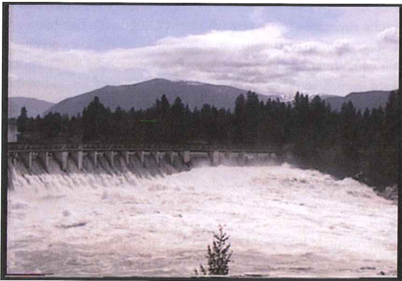
Photo 3 Main Dam at Thompson Falls, high flow (June 10, 2002, total river flow approximately 77,000 cfs)
