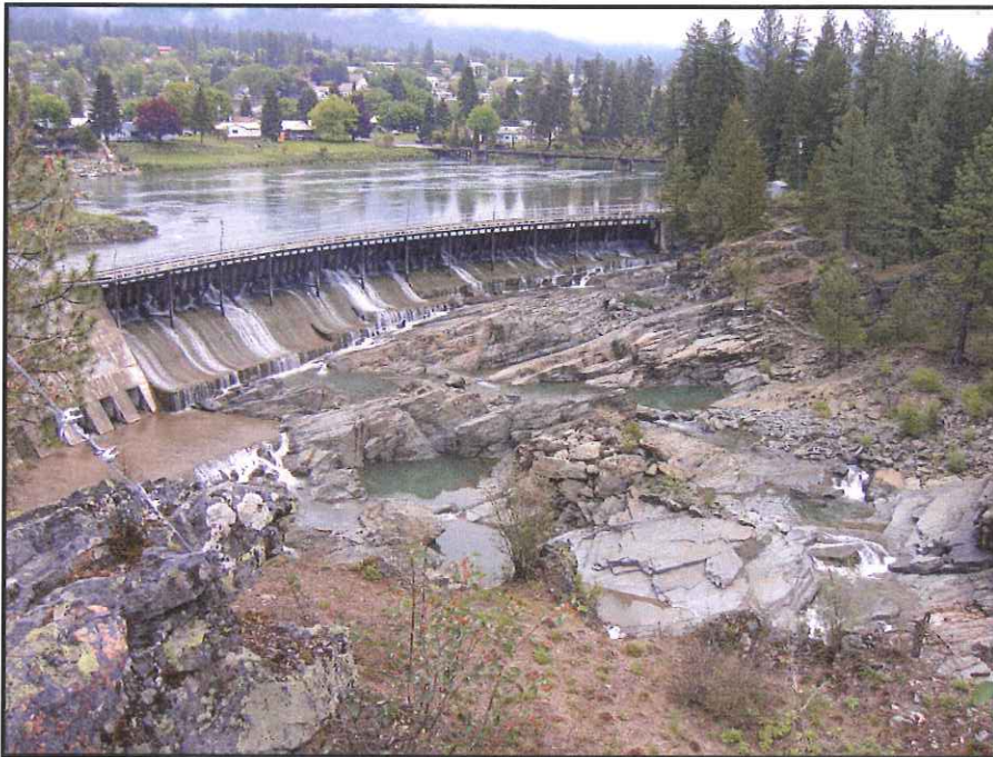
Photo 7 Dry Channel spillway, from above
