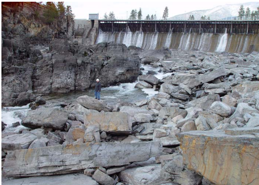
Figure 4 – Steep center thalweg and “falls” roughness.
